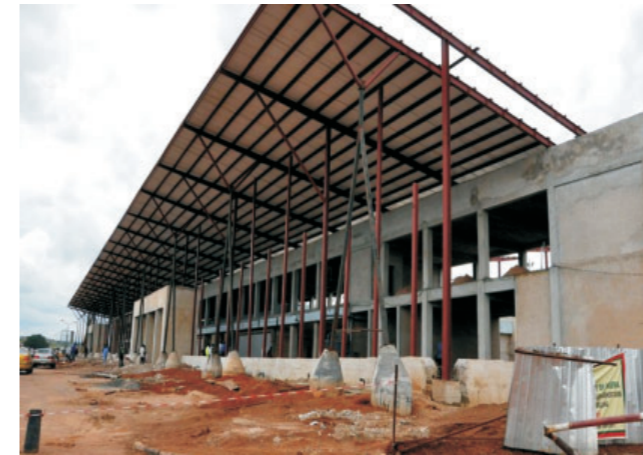
Enugu Airport terminal work in progress, October 2012
