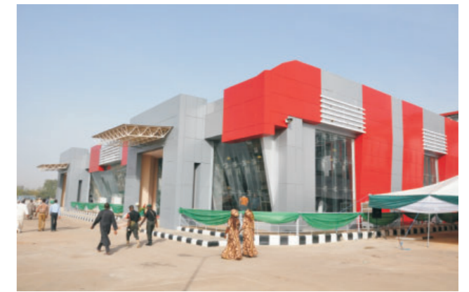
Mallam Aminu Kano International, newly remodelled International Terminal, March 2013
