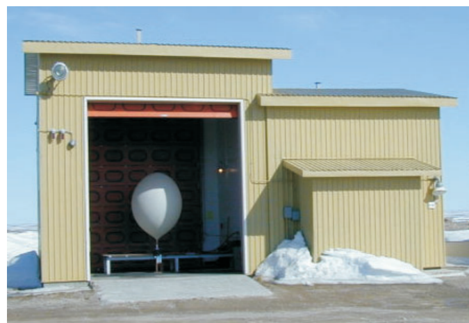
Hydrogen gas shed at Upper Air Station
