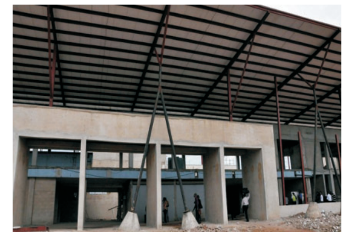
Enugu Airport old building disappearing as work progresses, February 2013
