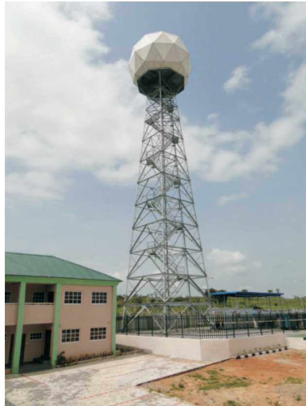
Doppler Weather Radar in Abuja
