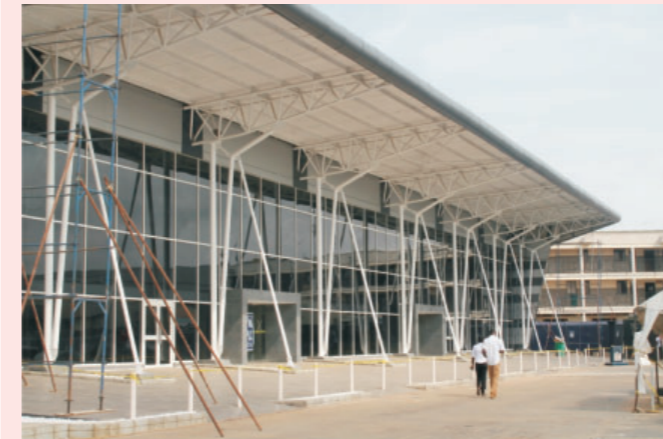
The new MMA Domestic Terminal 1 East Wing, March 2013 (below)
