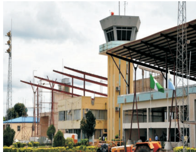
Enugu Airport terminal as remodeling commences, July 2012
