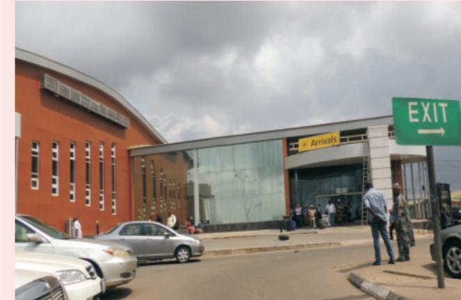
The new General Aviation Terminal, now named MMA Domestic
