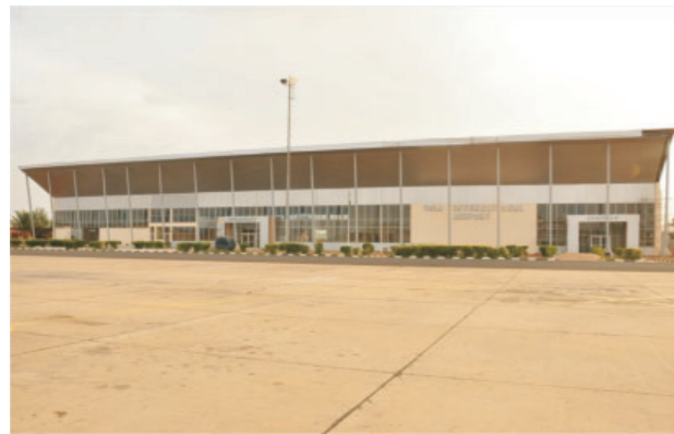
(iv) Remodeled Yola Airport Terminal nearing completion, April 2013
