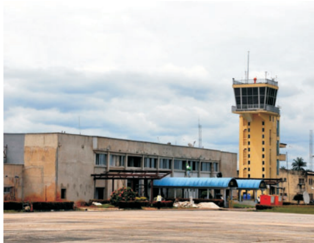
(i) Owerri terminal, January 2012
