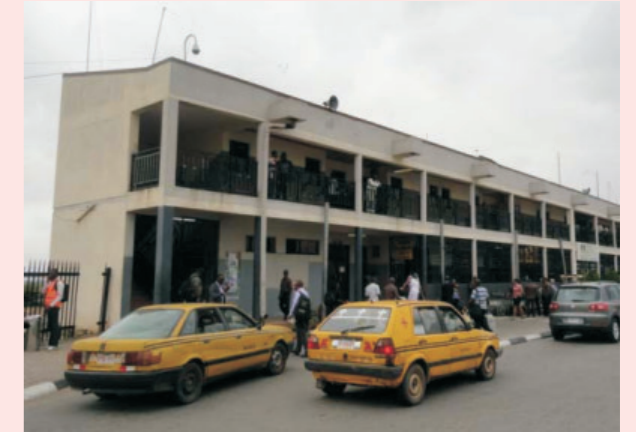
The old General Aviation Terminal, East Wing, January 2012 (below)
