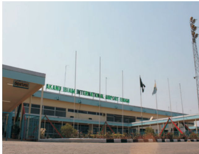
(ii) Enugu Airport Terminal, January 2012
