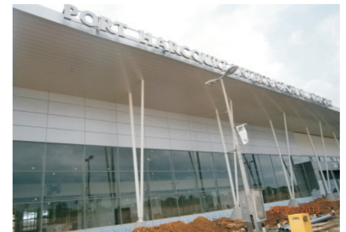
Port Harcourt International Airport Terminal, remodeling work in progress, April 2013
