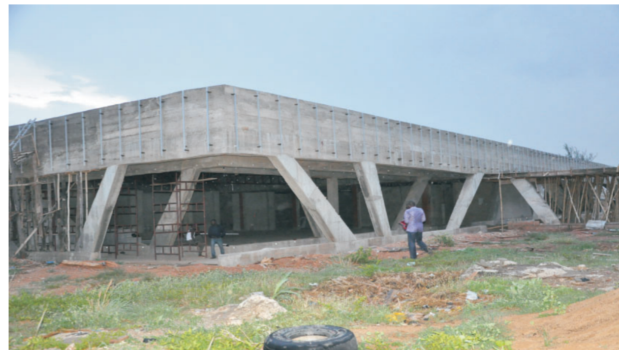
Kaduna Airport, remodeling work in progress, April 2013
