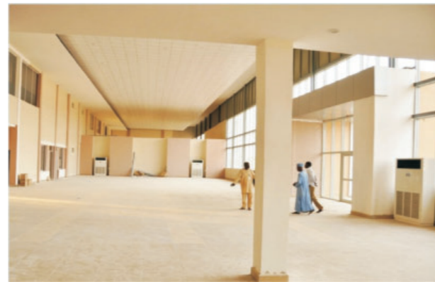
Remodeled Yola Airport Terminal, interior finishing touches, April 2013
