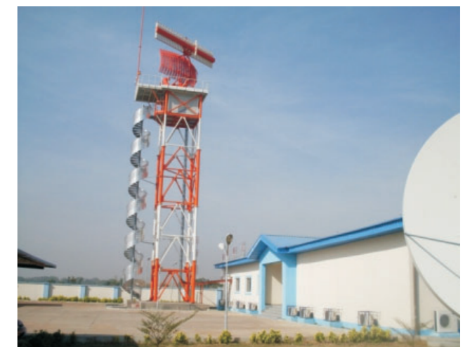
New Area Control Center, Abuja
