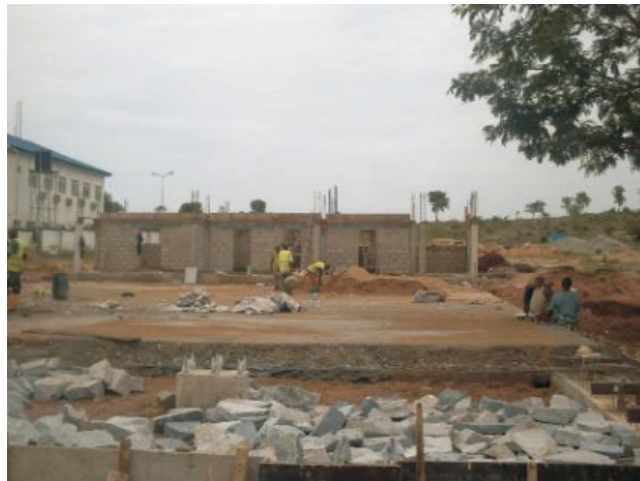
Pictures taken from Construction Site of above Project
