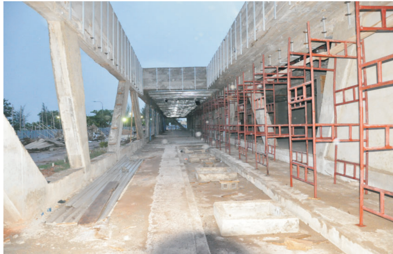
(vi) Kaduna Airport, remodeling work in progress, April 2013
