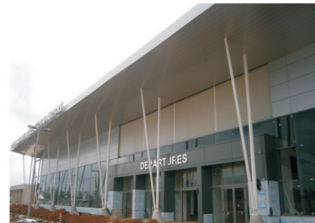
(iii) Port Harcourt International Airport Terminal, remodeling work in progress, April 2013
